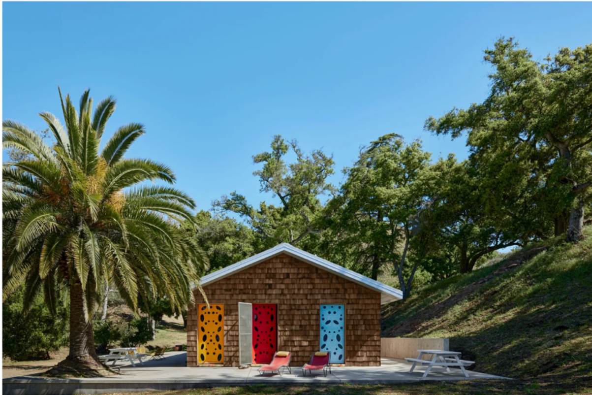
Colored panels set in the shingled exterior envelope pop against the verdant Malibu scenery.
