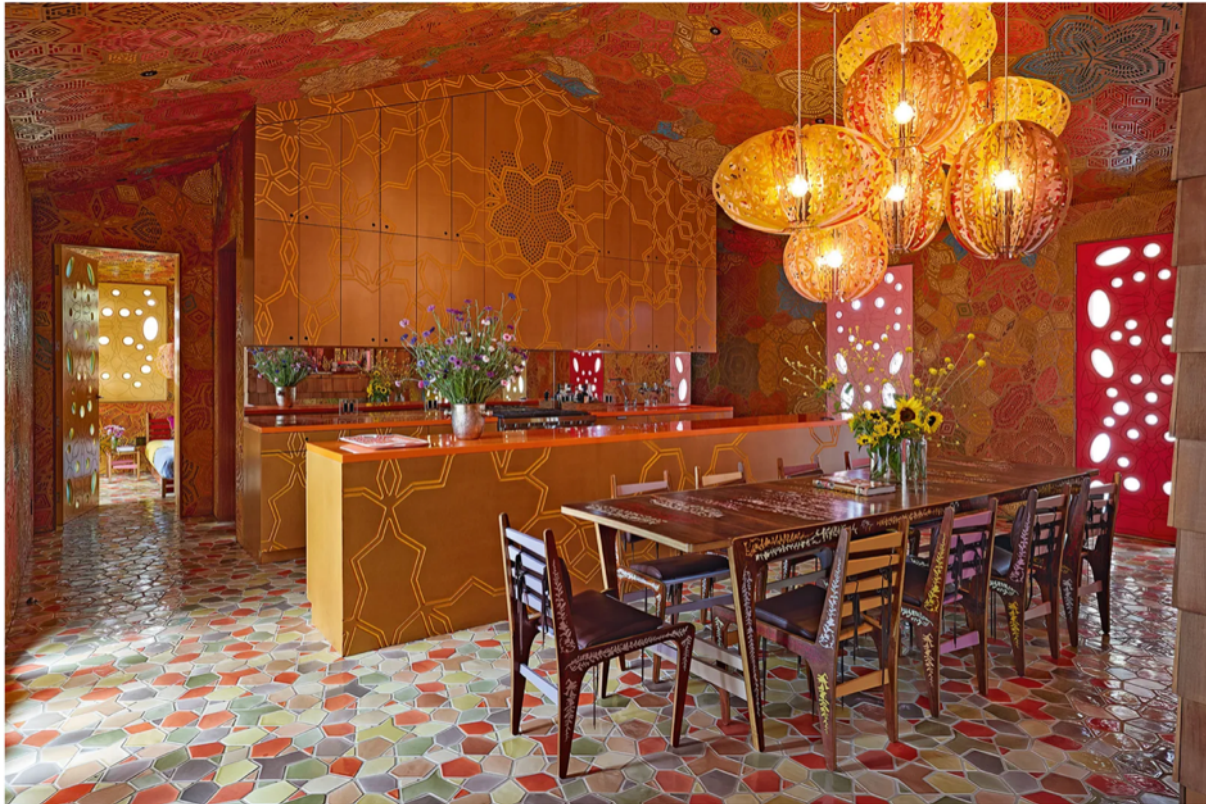
The kitchen has CNC cut/engraved MDF cabinetry panels and orange Corian countertops.
